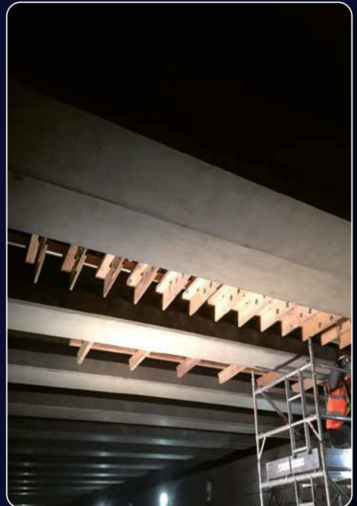
Figure 2 • The Completed Falsework
